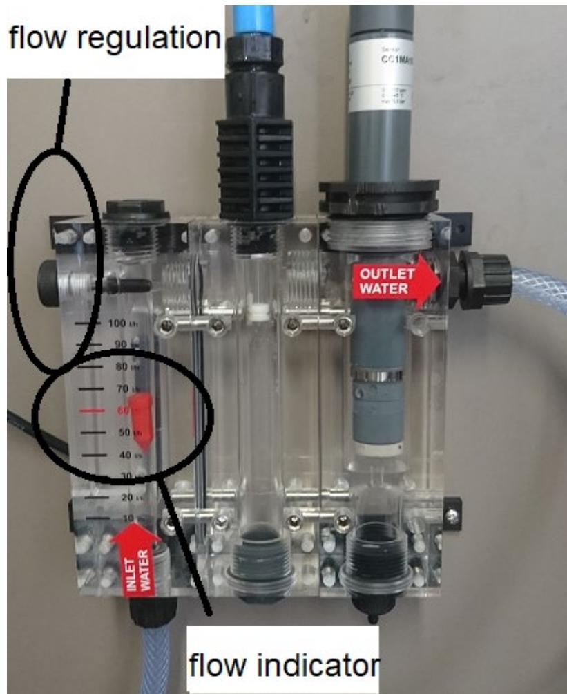
Switch on the electrolysis / dosing System. The CL reading will increase slowly and will be stable after some minutes.
